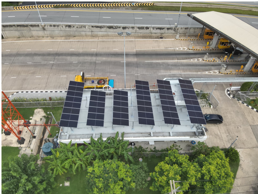
"Solar Power System Installation on Toll Building Rooftop of the Udon Rattaya Expressway" Project
