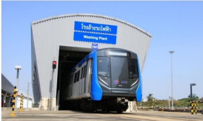
Water Recycling System Project for Train Washing Plants
