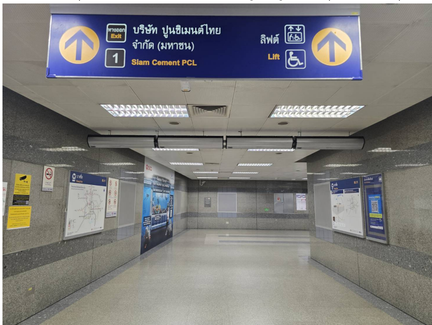
Project to install air curtains at entrances and exits in the MRT Blue Line Project (Phase 2)
