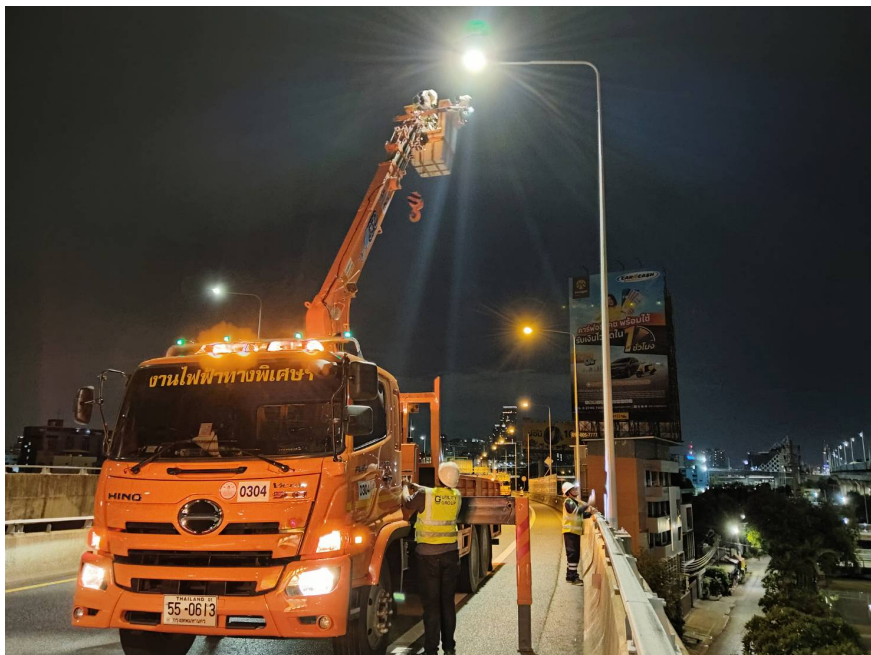
LED Lighting Replacement Project on the Si Rat Expressway (SES)
