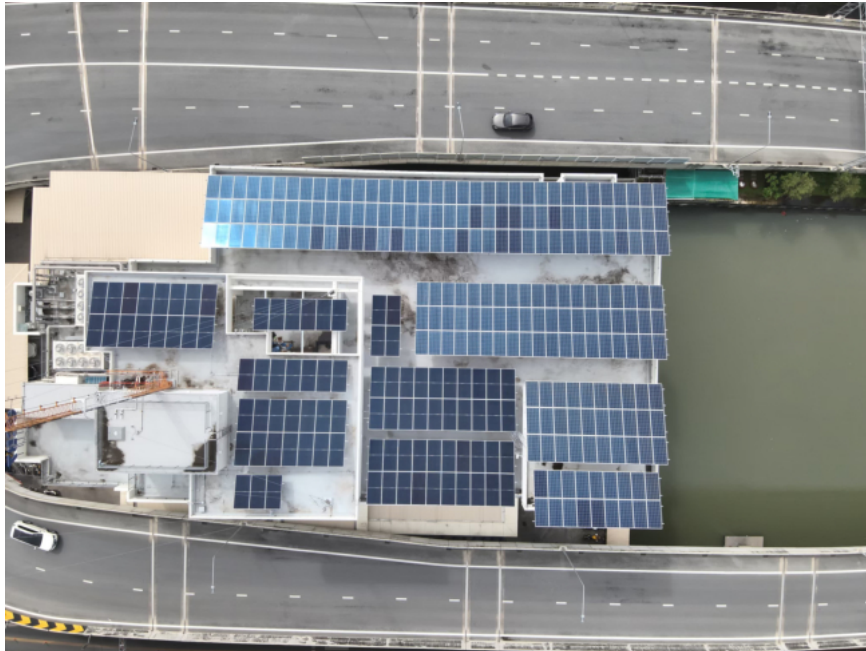
"Solar Power System Installation at Prachin Rattaya Control Center" Project
