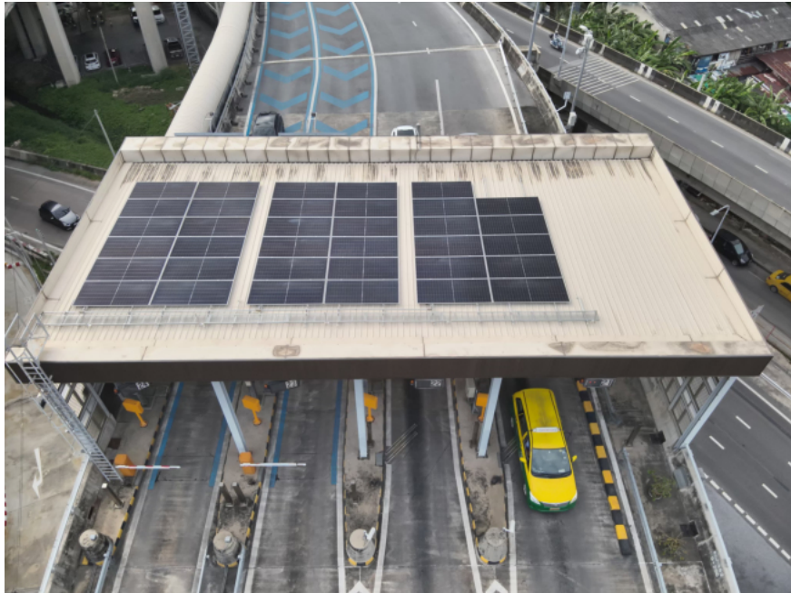
"Solar Power System Installation on Toll Building Rooftop of the Si Rat Expressway" Project
