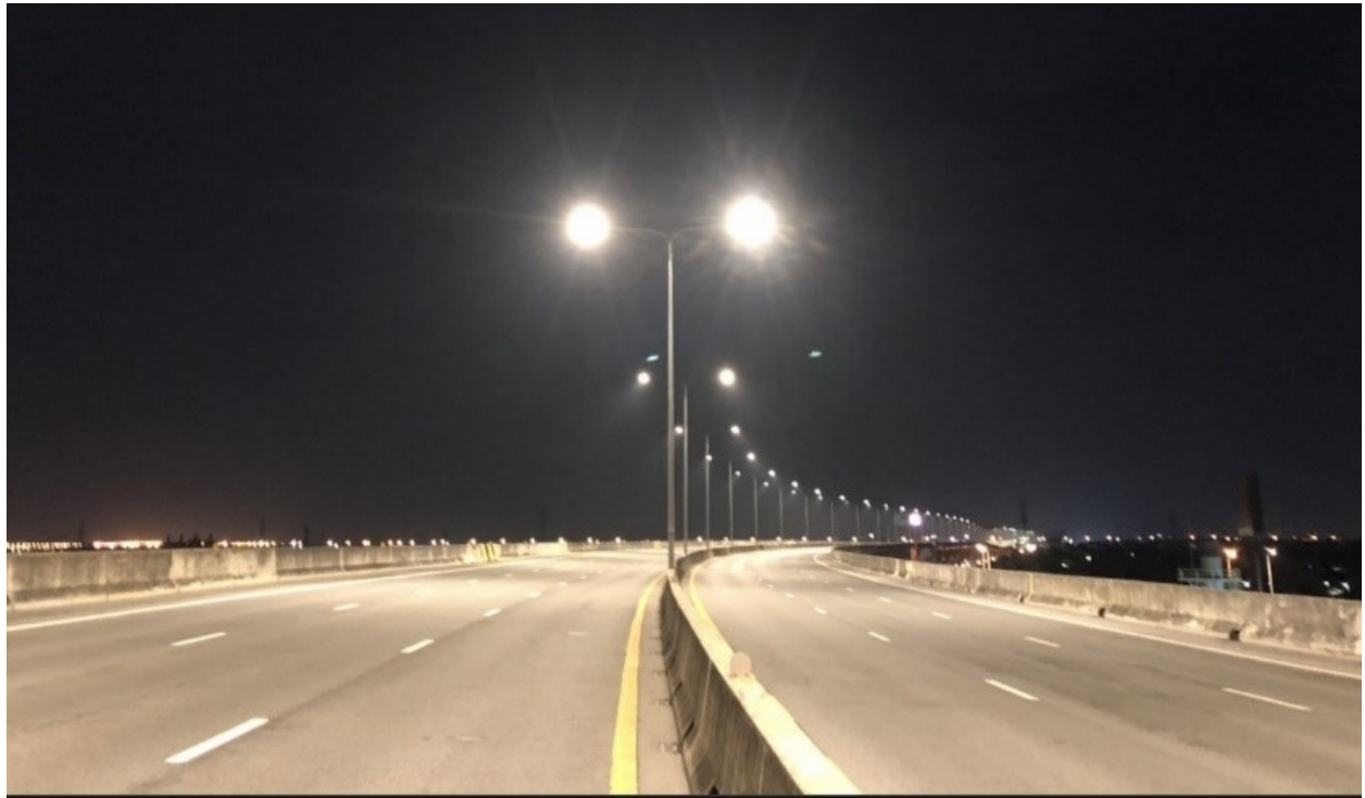
Replacement of HPS lamps with LED lamps along the Mainline of the Prachinrat Expressway (SOE)
