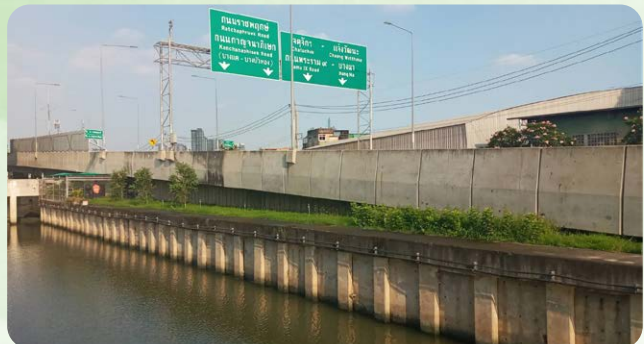
Retaining Wall along Sung Canal
