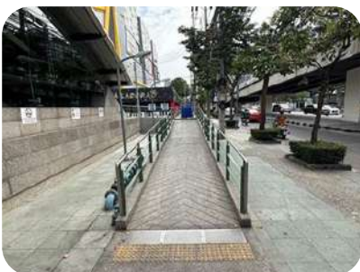
Ramp for wheelchair users
