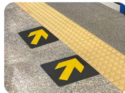
Tactile surface indicating changes in level
