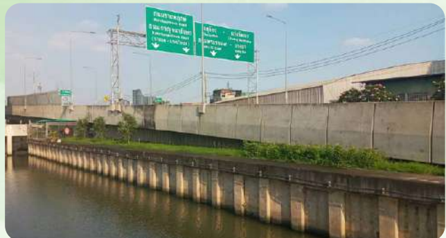
Retaining Wall along Sung Canal
