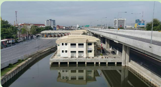
Prachin Ratthaya Expressway Control Center
