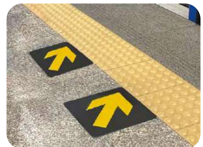
Tactile surface indicating changes in level
