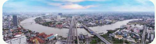
Bridge Crossing the Conservation Canal Construction project
